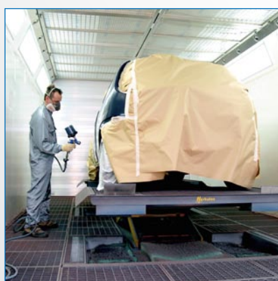
The lift HLS as in-ground installation in the spray booth.
